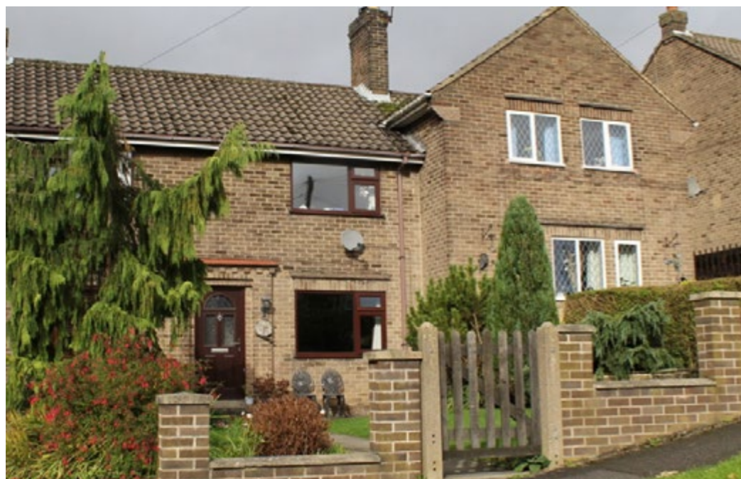
Left: Front-projecting gables, brick boundaries and soldier coursing for window details all mark out this more modern housing in Nightingale Close.
