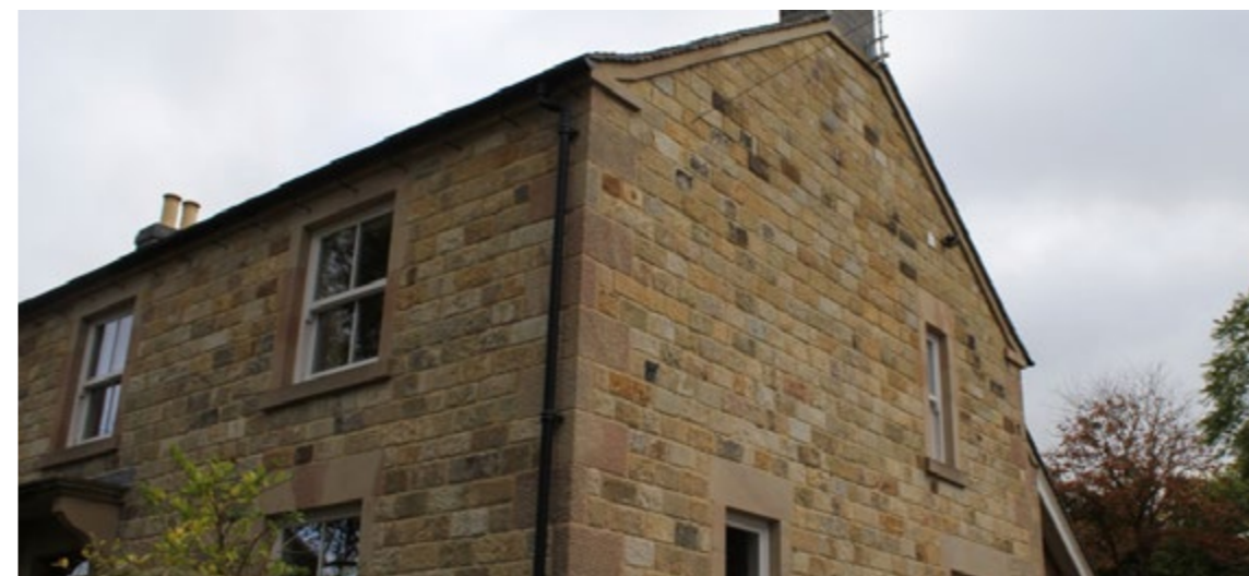
Right: Newer properties using a sympathetic building material and detailing, with flat laid blocks and sash windows.
