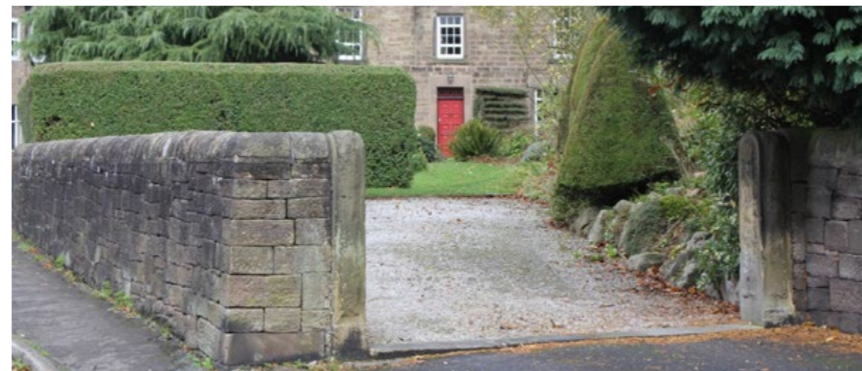
Right: Lea Mills, with dressed and formed blocks, making the boundaries here more industrial and formal.
