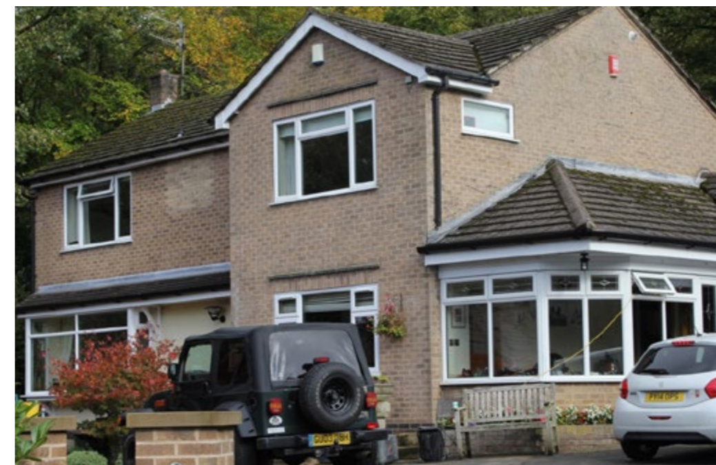
Right: White uPVC and barge boarding / soffits combined with a buff brick are all out of character with the older parts of the area.
