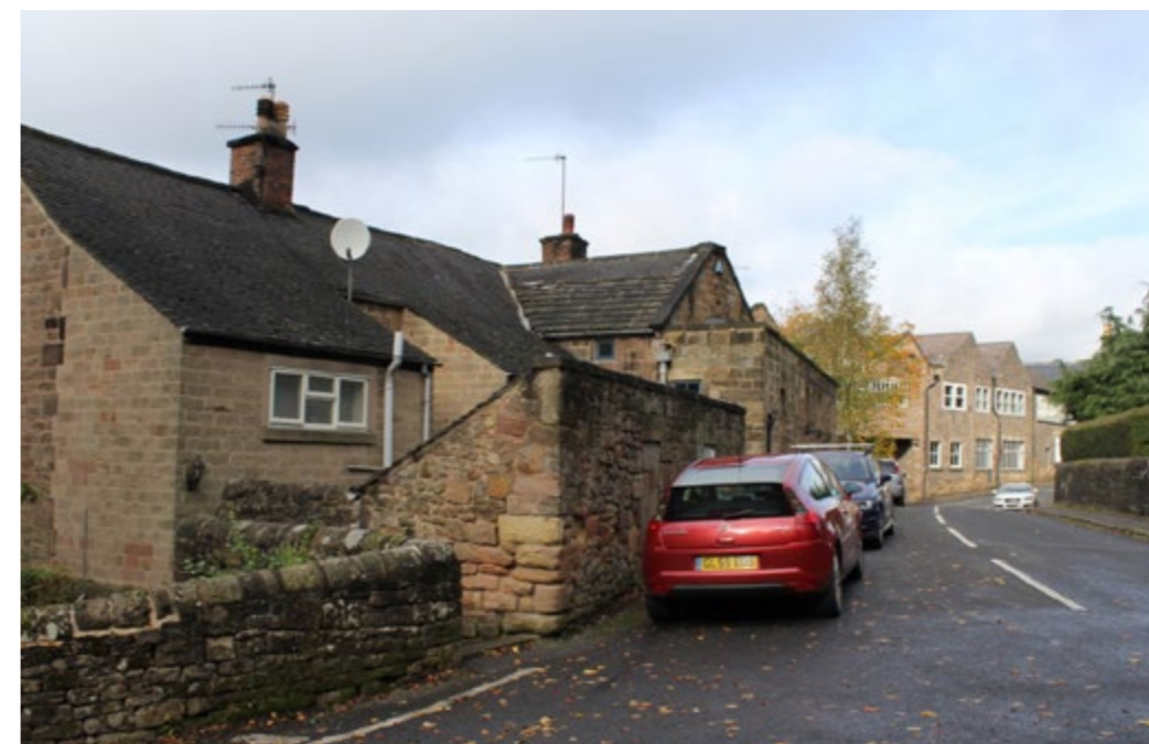
Right: Workers cottages close to the street create a feeling of enclosure in Lea Mills.
