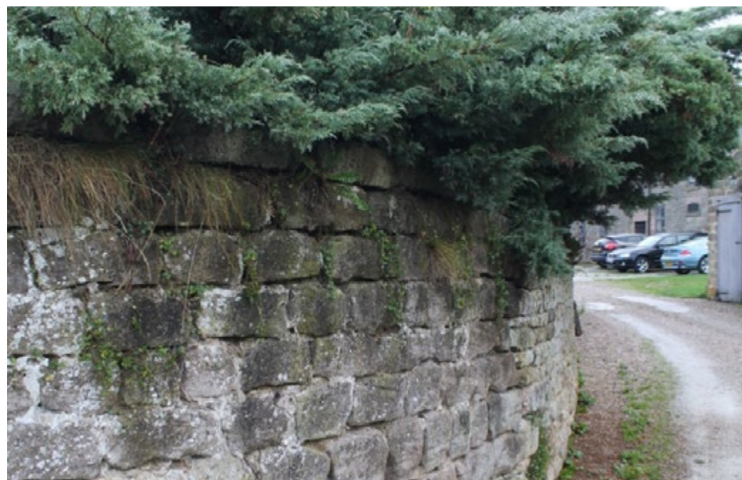
Left: Flat-laid stone block walls are typical of the area, as in here at Dethick.
