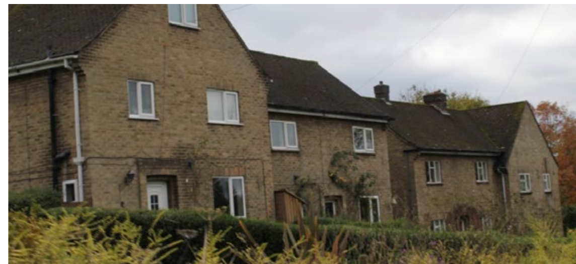
Right: On newer development, buff brick has been used, as have front-projecting gables for the roofs. These are not in character with the village.
