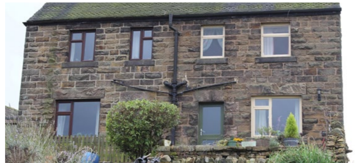
Right: Gritstone blocks, with stone lintels for windows and doors are the most common materials in the village.
