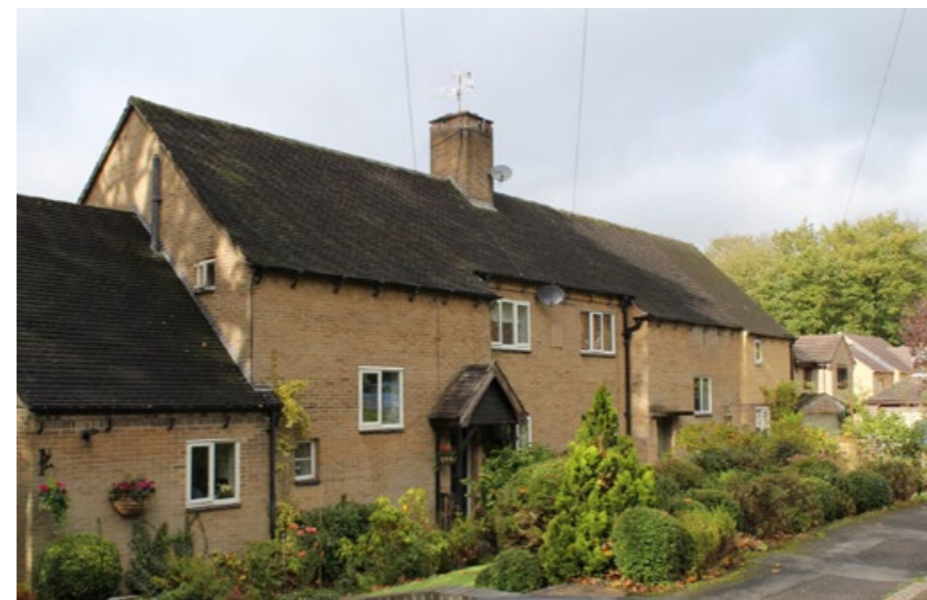
Right: Hollins Wood Close, another late addition to the area, with a more estate like design of regular footpaths and low ornamental planting.
